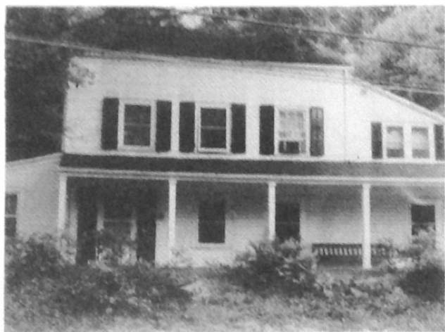
REAR VIEW - THOMAS DODGE HOUSE This view shows small leaded glass windows in upper storey. Thomas Dodge was the son of early settler, Robert Dodge.
